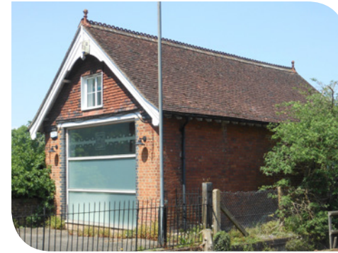
Clay tile roofs with decorative ridges
