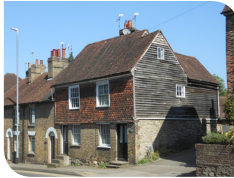
Tile-hanging and weatherboarding
