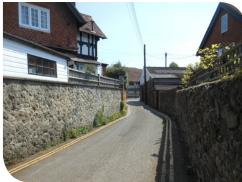
Kentish Ragstone walls
